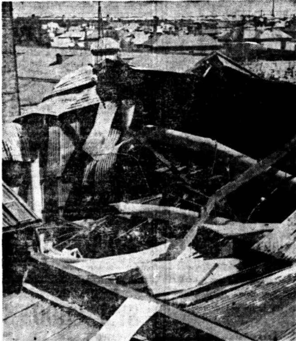
A GENERAL VIEW of the damage caused by the fire at the factory of J. W. McGregor & Sons, Ltd., Thebarton. Damage was estimated at £1,000.
