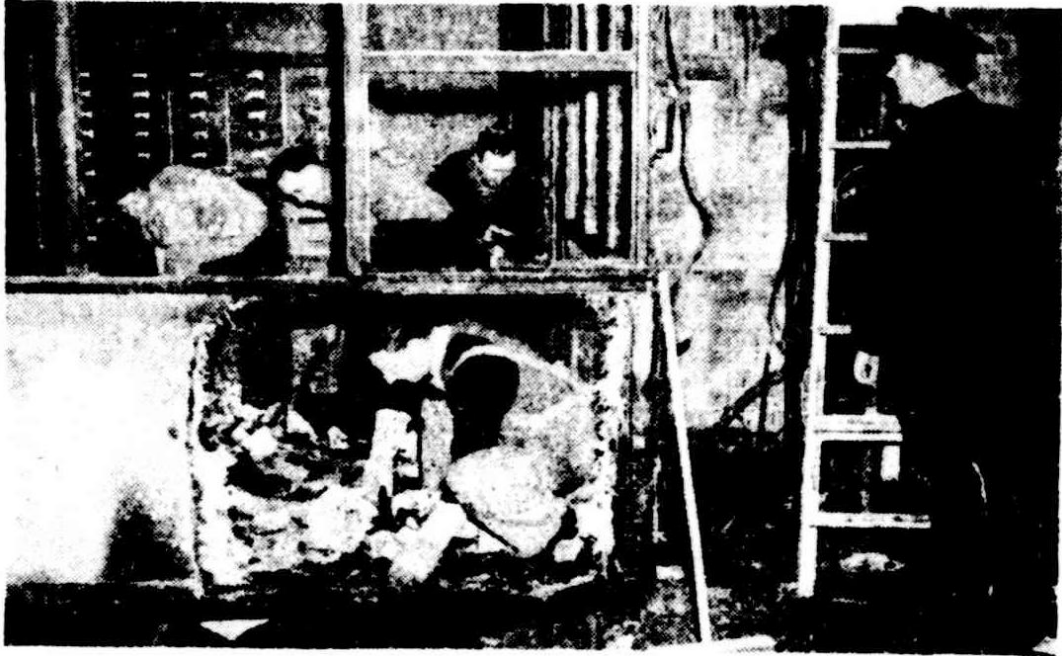
Clearing up the premises of Charles Richardson and Sons, Southwark, after heavy damage had been done to the premises by fire yesterday morning.
