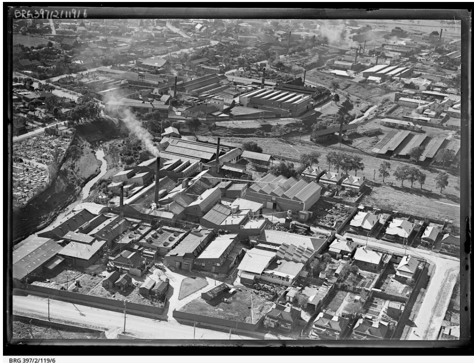
State Library of South Australia - Item 06: Torrensides Woollen Mills, Thebarton. [BRG 397/2/119/6], Aerial photograph of Thebarton, looking north east. South Road and the Torrensides Woollen Mills are in the foreground. The River Torrens runs from the left of the image through the centre of the view. Hindmarsh is in the background. 1938. Photographer, Smith, D. Darian. Part of D. Darian Smith and Thebarton Collection.
