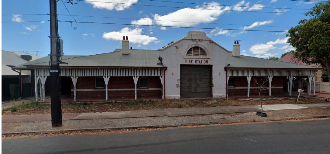
Thebarton Fire Station 2024 Google Maps
